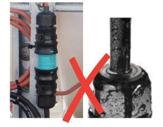
Place connector horizontal in a way that leads draining water away from cable gland.
