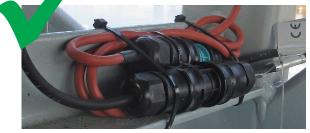
Cables may not dangle in the wind as they can be pulled out of the cable inlet, and open for water ingress.
